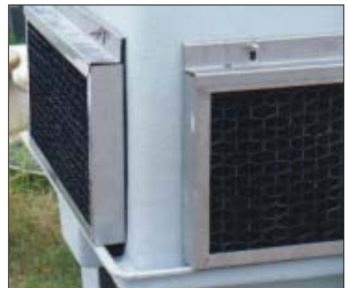
▲ Access panels and anti-splash louvres are easy to remove. Note the fixings the minimum number of fixings.
