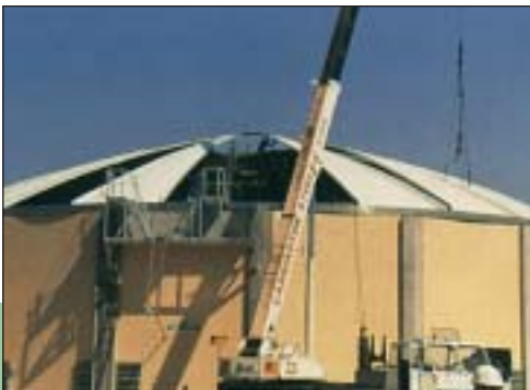
▲ Installing a 30 m self-supporting fibreglass dome for odour control plant.
