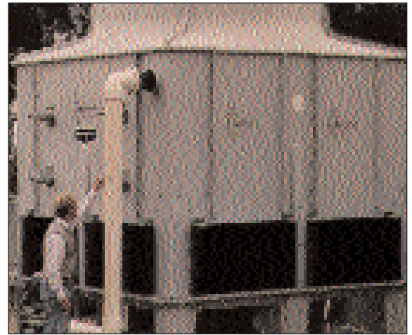
▲ Large access panels make servicing easy
