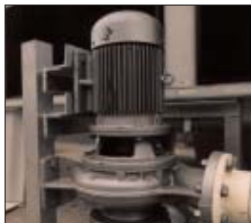
▲ Motors, drives, pumps are all located externally for ease of operator access. No need to enter confined spaces to adjust belts and so on.
