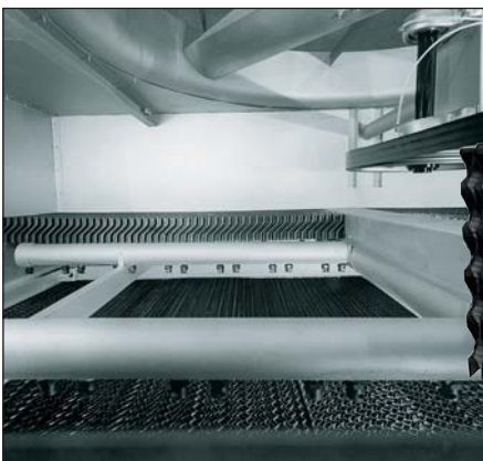
The water distribution system is made of Class E PVC pipe and ABS plastic water diffusers.
