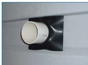
The water distribution system is made of Class E PVC pipe and ABS plastic water diffusers.
