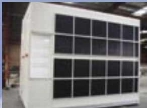
Australian Institute of Sport Air Handling Unit 12,000 L/s with Hot/Cold Water coils and return air bypass
