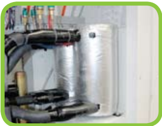
De-super heater option for free hot water heating
