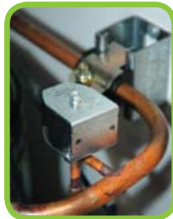
Hot gas de-ice solenoid (centre) pipe support (top right)
