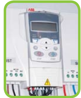
Variable Speed Drives control fan speeds, reduce commissioning time and provide additional electronic protection for fans and motors.
